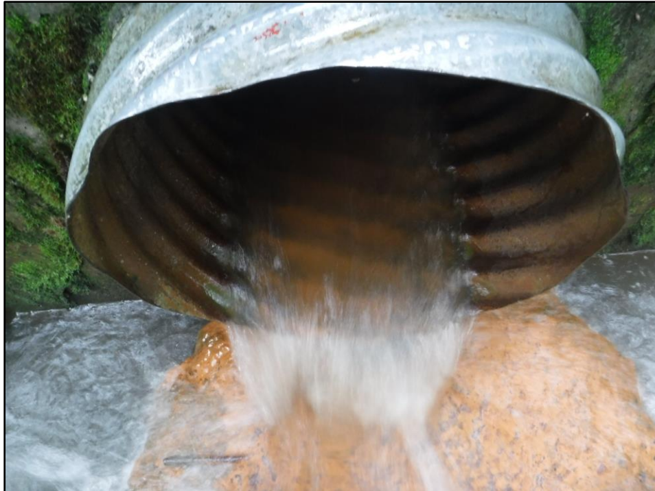
Photograph 10. Outfall SWM10 (525-2), Eagle Street at Chester Creek.
