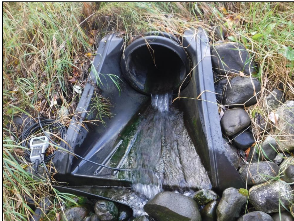
Photograph 2. Outfall SWM02 (847-1), Home Depot on Abbott Road.
