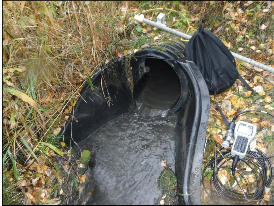
Photograph 1. Outfall SWM01 (1040-3), Ridgemont Drive.
